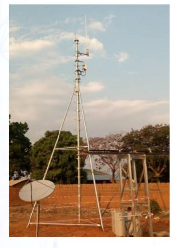
TOWER: 10 m, 12m BTS: OC2G 1 TRX @ 630 MW ANTENNA: 10 dBi Omni Exclusively solar powered VSAT BACKHAUL 24 HOURS AVERAGE POWER CONSUMPTION: 64W COVERAGE RADIUS: Up to 2 km POPULATIONS COVERED: Approx.2500 inhabitants
